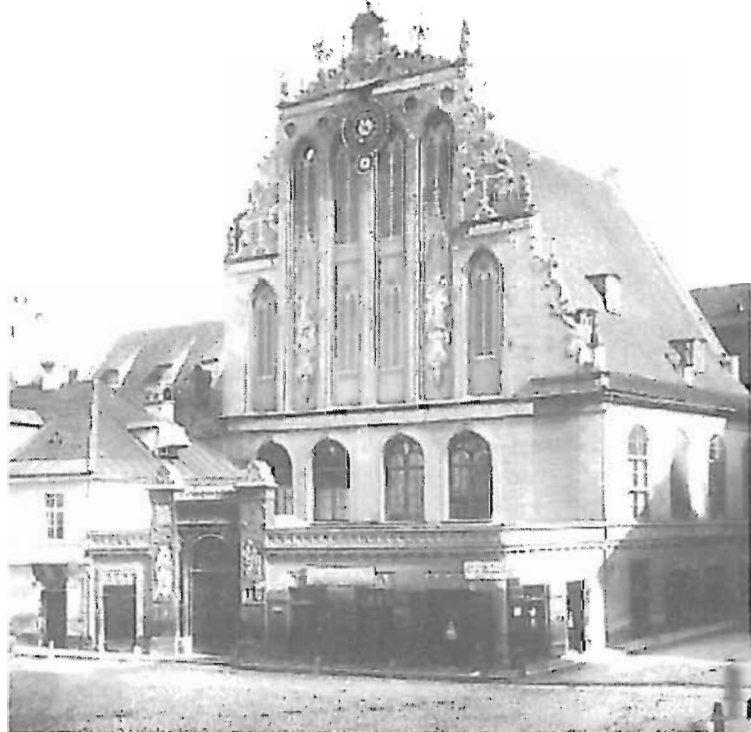
Restoration of the Blackheads House.
