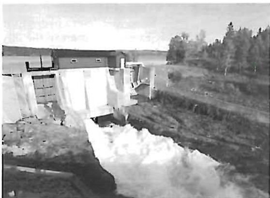
Juvvuln hydro power station (in Sweden)
