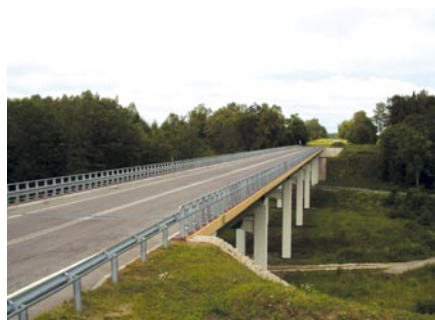
Renovated bridge on 'Berlinka' road
