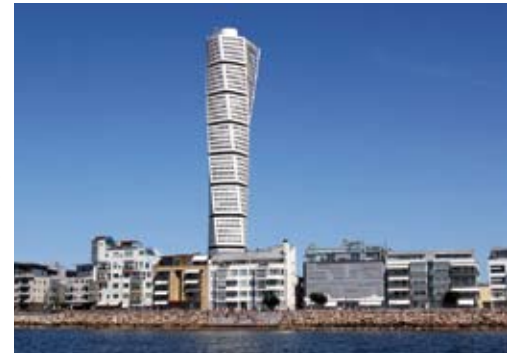
City of Malmö from the sea with the sustainable housing area of the Western harbour and the Turning Torso.
