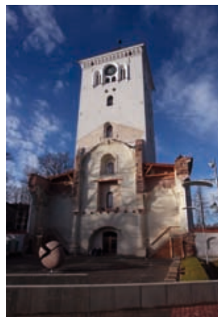
Recently renovated St. Trinity Church tower
