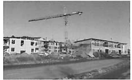
Construction has started at Mäkikaivo
