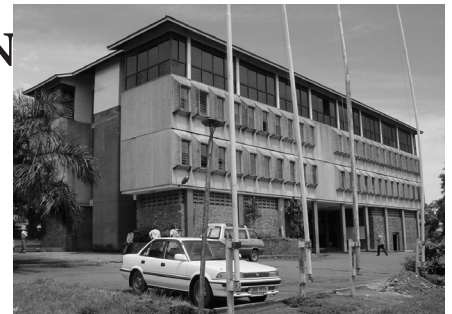
The LVRLAC Secretariat is located in the same building where the City Authorities have their premises
