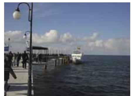
The view of new pier in Międzyzdroje
