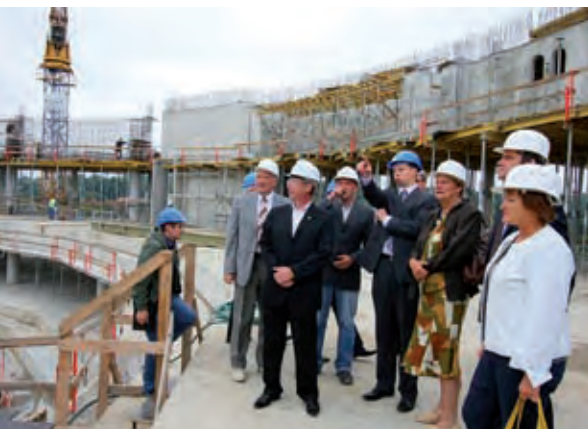
Kaunas City Sports and Entertainment Arena is successfully under construction, the value of which is 50 million EUR. EU funds are expected to contribute nearly 15 million EUR.
