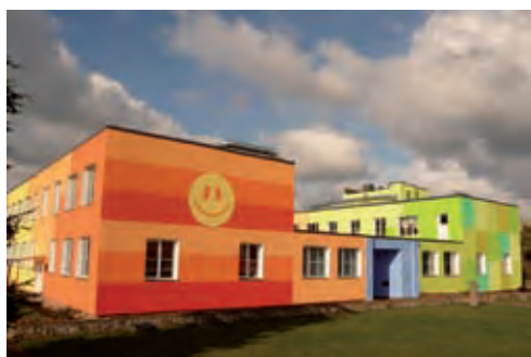
The main goal of the improvement of energy efficiency in municipal buildings is to save up the costs for heating and decrease the carbon emission impact.
