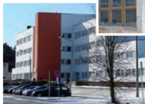
Jēkabpils district central hospital before the renovation (up on right hand side) and after - with new windows, the roof and insulation
