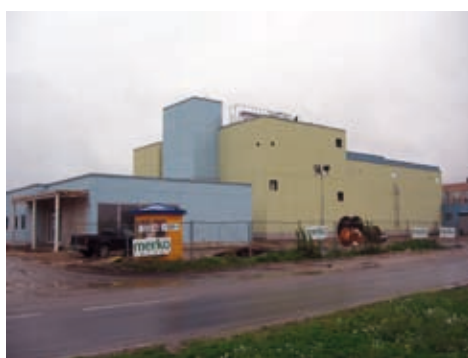
The water-treatment plant in Narva was built from scratch and now it strives for new ambitious projects.
