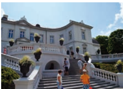
The Counts Tiškevičiai Palace, the home of the Amber Museum which is famous not only in the country but far beyond its boundaries, undergoes the renovation.
