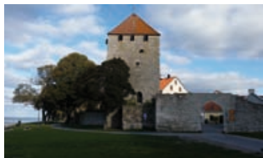
The one of the oldest parts of the ring wall called "Krutttornet".
