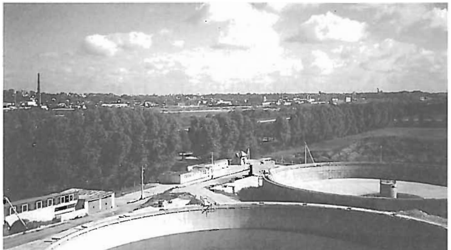
Sewage treatment plant in Kaunas is scheduled to be in full operation in May 1999.
